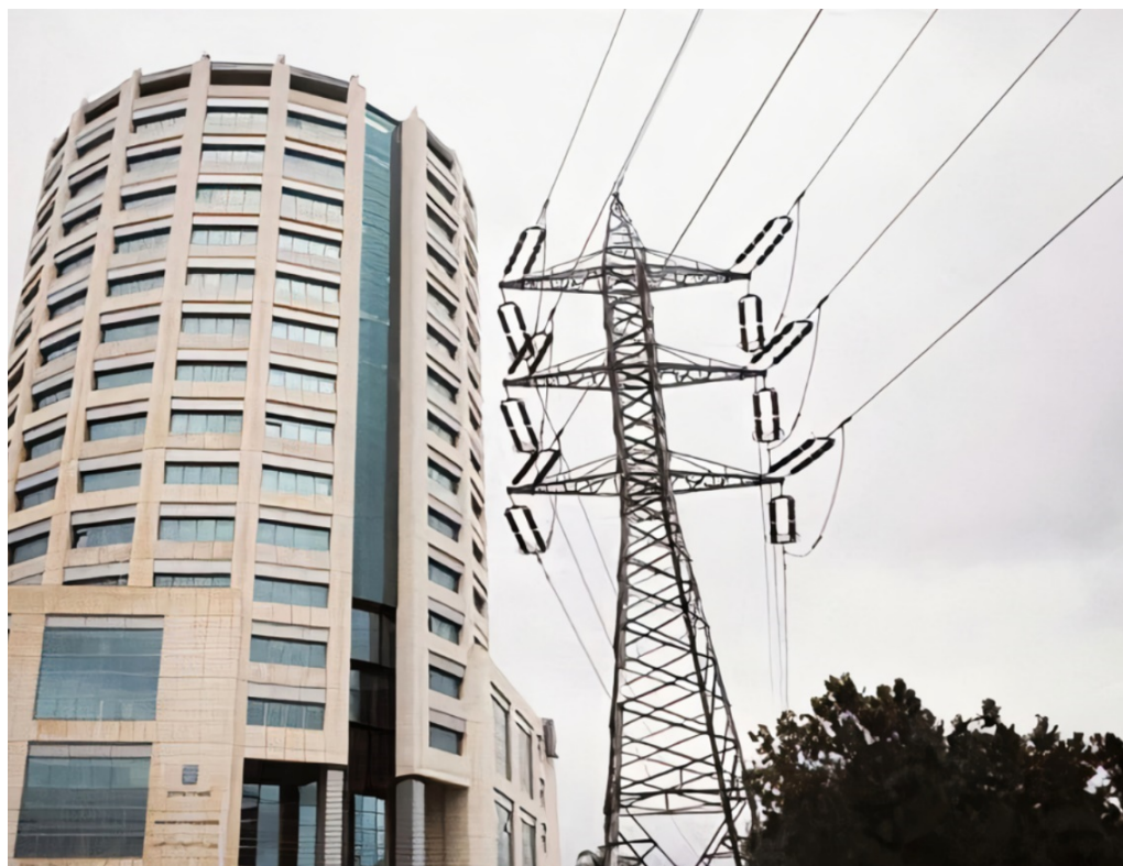
Figure 1. Office building under study and nearby high-voltage power line.
